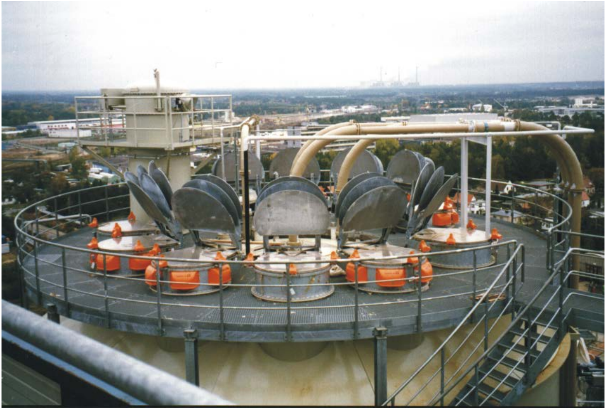
Figure 7-2. Explosion doors with integral vacuum breakers to avoid an inadmissibly
