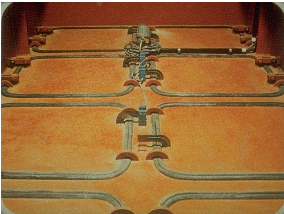
Figure 5-9. Explosion panels supported by rubber mouldings; panels restrained by cables from flying away /14/
