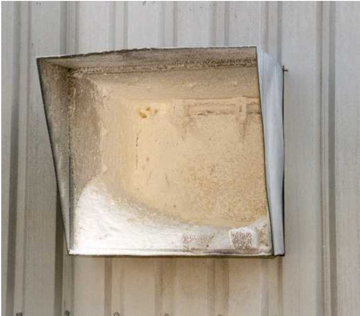
Figure 19-1. This explosion door needs immediately maintenance to avoid severe consequences in case of an explosion
