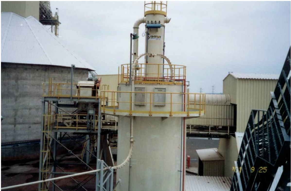
Figure 6-17. Silo vented on the side
