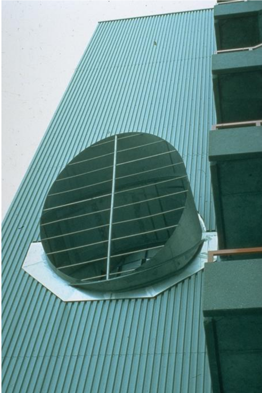
Figure 9-12. Vent duct angled downward slightly with additional mesh
