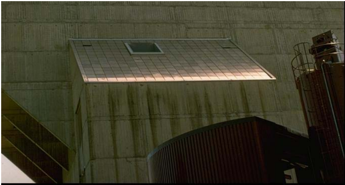
Figure 4-1. Venting of enclosure through the roof
