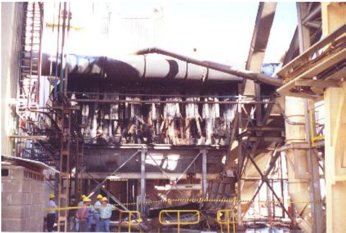
Figure 6-3. Consequences of no installing isolation systems
