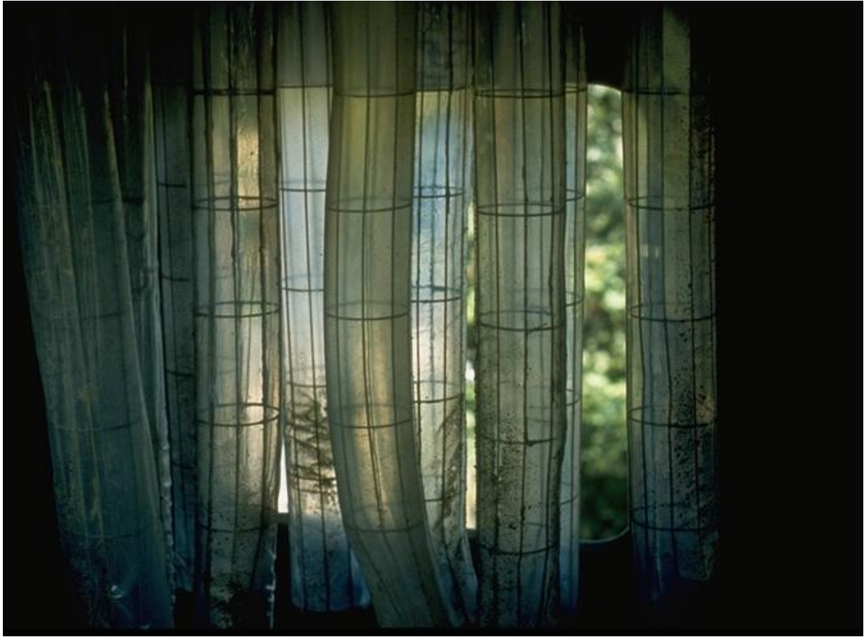
Figure 6-12. Filter hoses obstructing vent area
