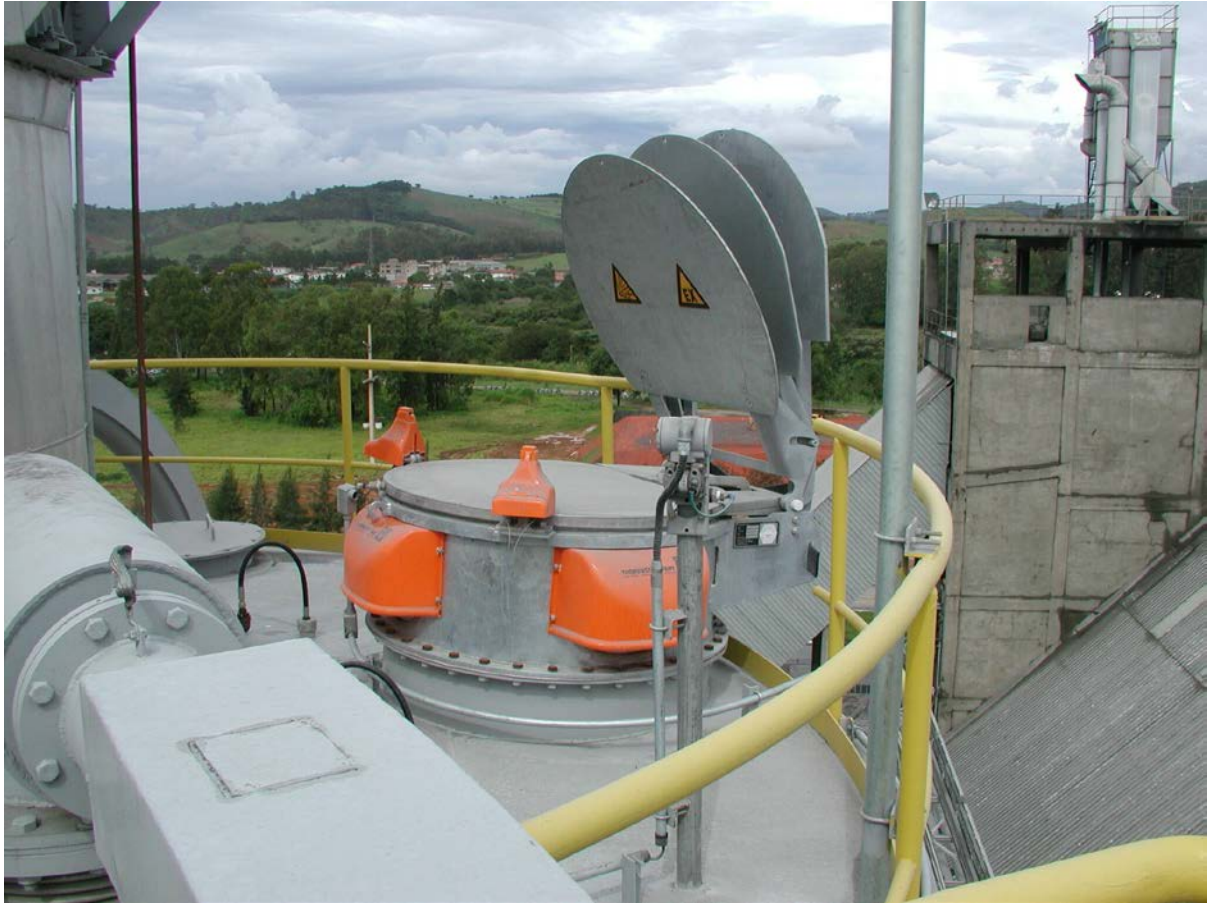
Figure 5-22. Silo roof: correct protected with an explosion door and integrated vacuum breakers /15/
