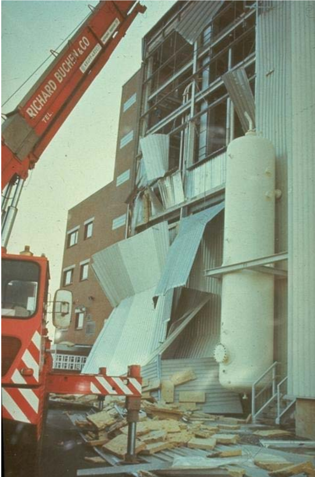
Figure 4-2. Facade covering of a production building after a dust explosion
