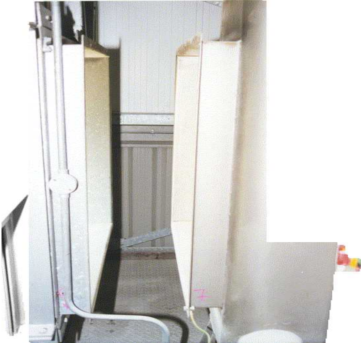
Figure 9-18. Missing rubber compensator for the connection between protected vessel and vent duct
