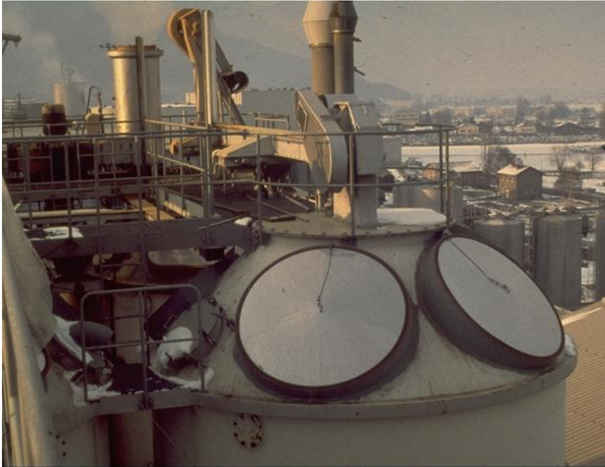
Figure 6-16. Roof of a silo, approximately 2/3 of roof used as vent area
