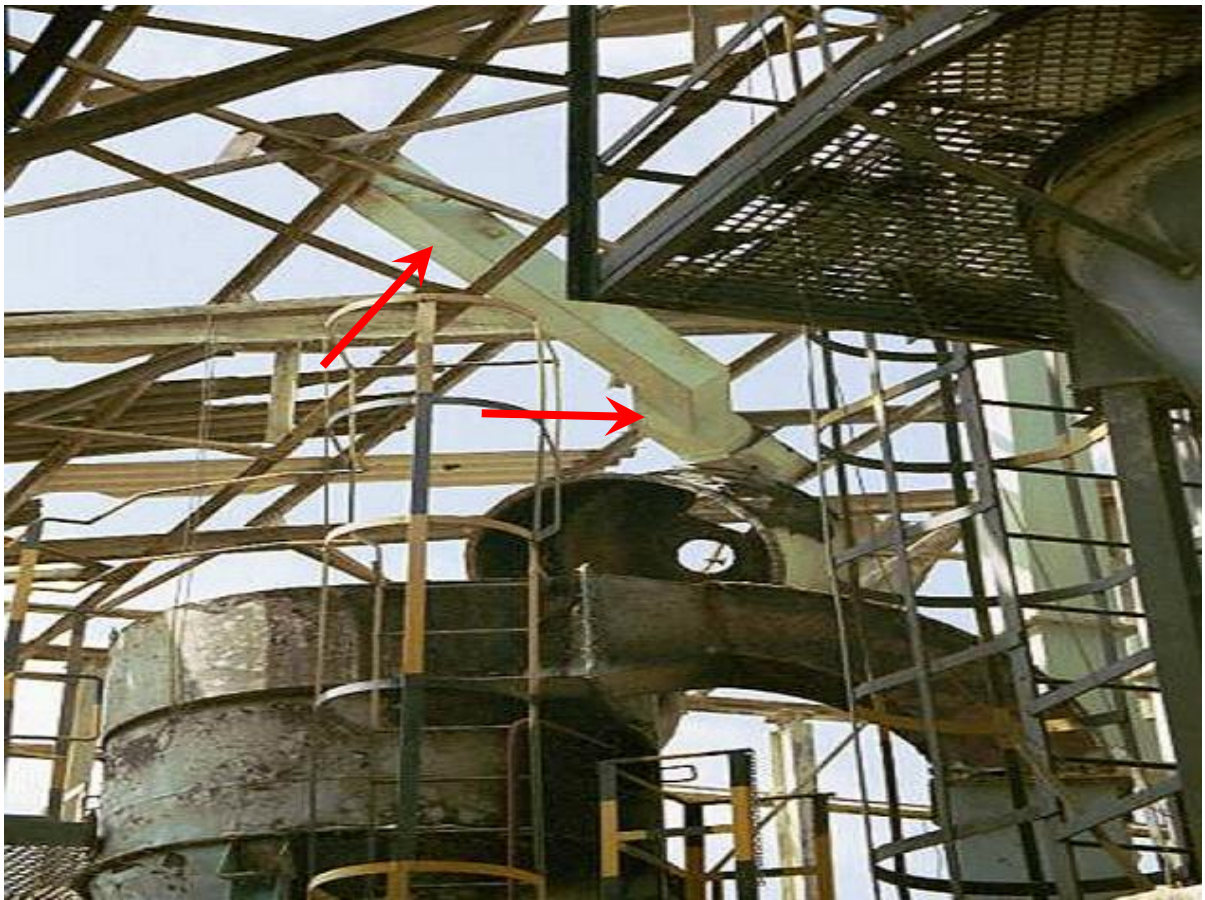
Figure 9-1. Consequences of a bad design of vent duct
