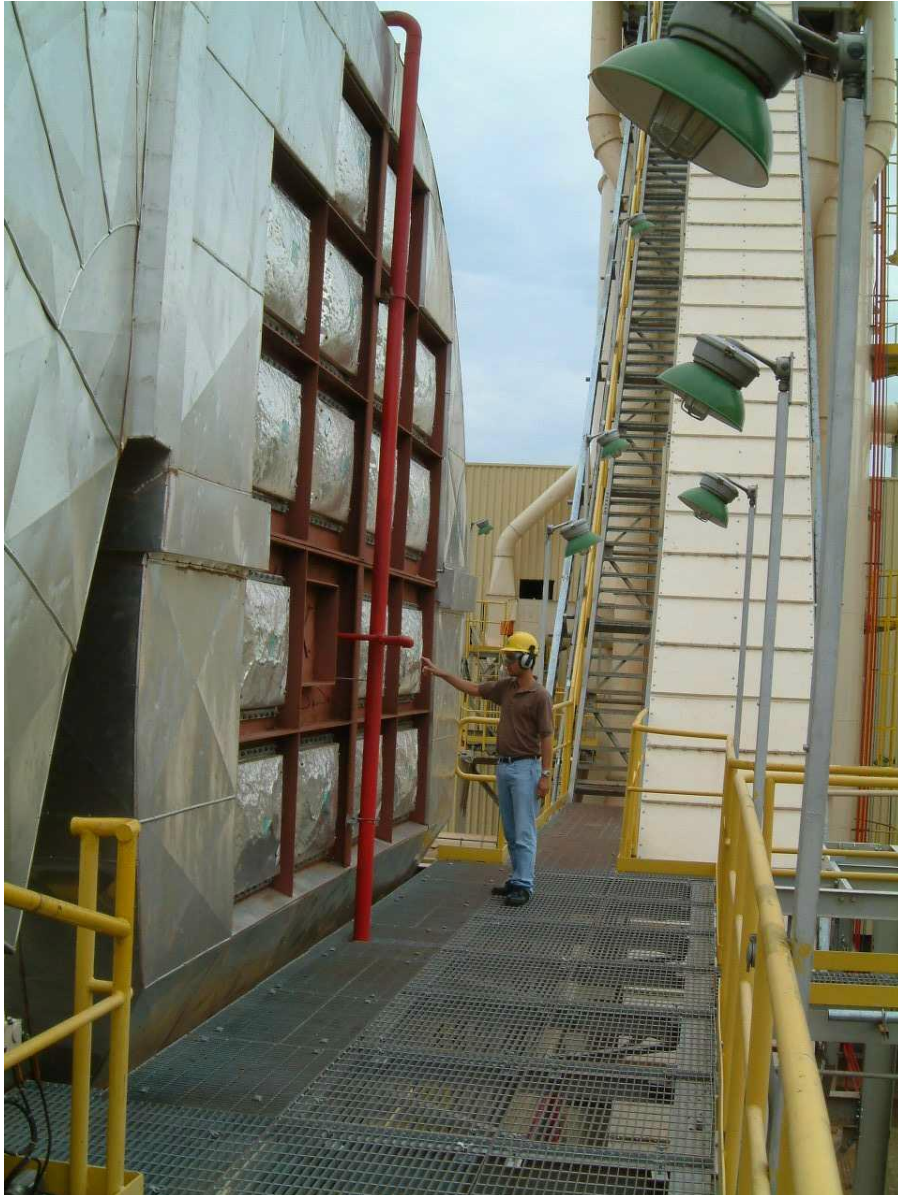
Figure 3-5. Endangerment of personnel by poorly placed vent areas
